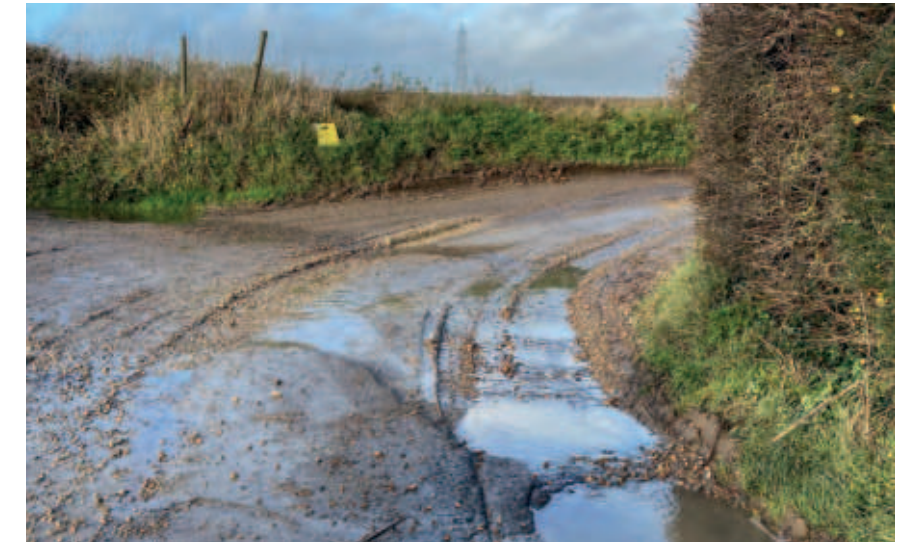
Tackling localised flooding
