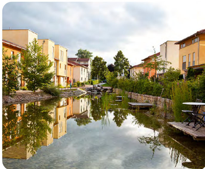
SuDS can create multi-functional spaces which contribute to human, ecological and environmental amenity.
